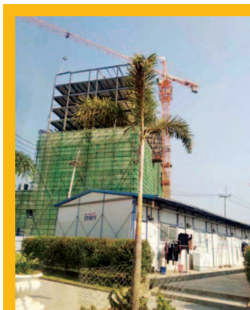
Advanced construction at Shwe Kokko February 2020
