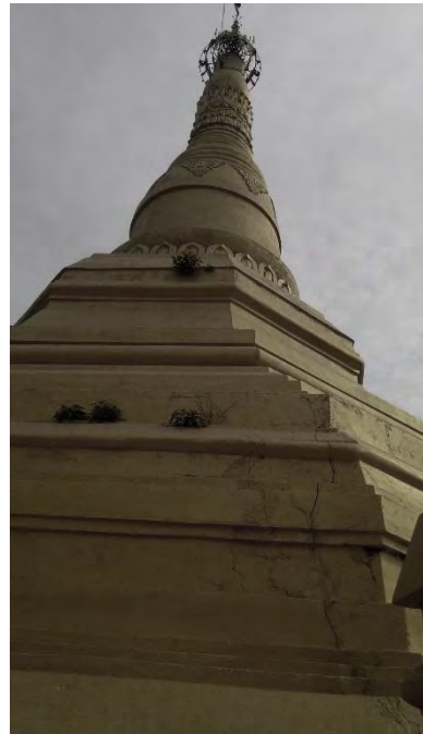
Figure 39: Historical artefact has visible cracks which is believed to be caused by stone mining
